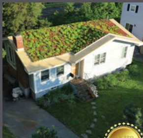
Private Residence Winchester, MA Extensive Green Roof
