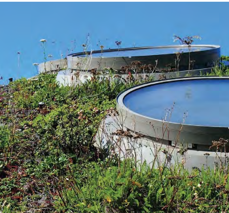
CALIFORNIA ACADEMY OF SCIENCES GREEN ROOF
