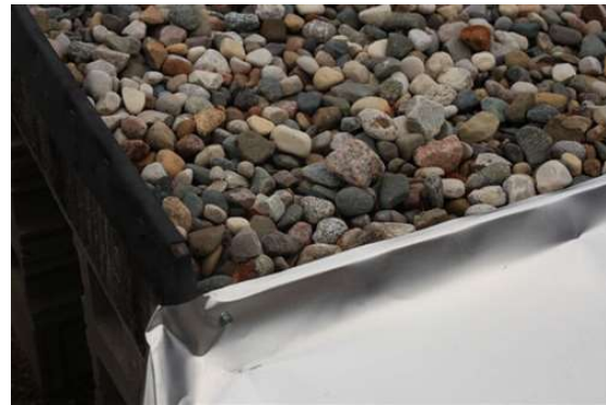
2F. Gravel ballast
